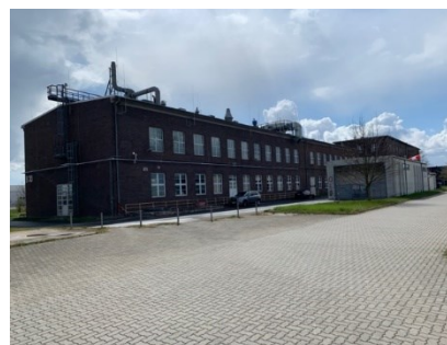
IOLITEC @ Schkopau, Germany.
