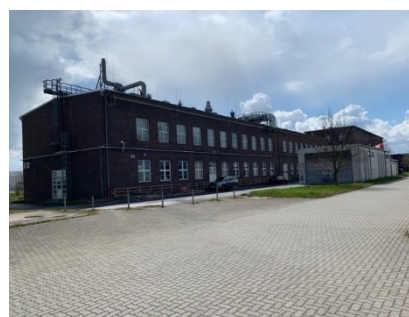
IOLITEC @ Schkopau, Germany
